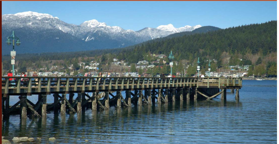
Pier at Rocky Point Park, Port Moody
